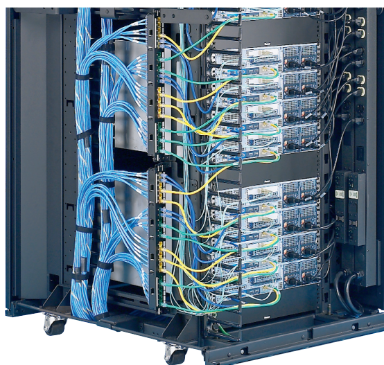
Figure 9. Cabinet Vertical Mount Patch Panel
