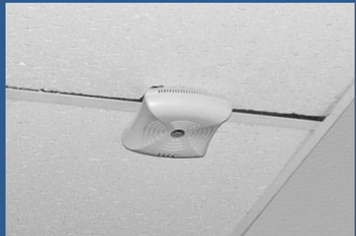
These types of openings in the ceiling tile are undesirable in a healthcare environment.
