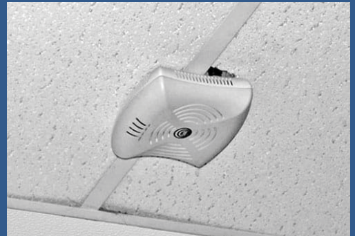
Examples of intrusion into the above-ceiling space
