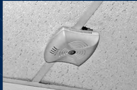
Examples of intrusion into the above-ceiling space
