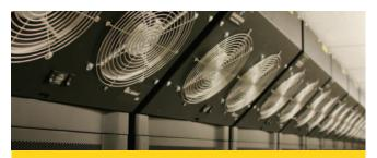
"The Liebert XDV units have a low profile, allowing them to fit on top of the racks without changing the ceiling height or requiring major modifications to the new ceiling."
