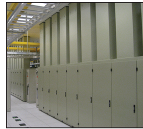
Belden Passive Chimney Containment is available with Through-Ceiling chimneys and Against-Ceiling chimneys for in-row heat extraction from cabinets.
